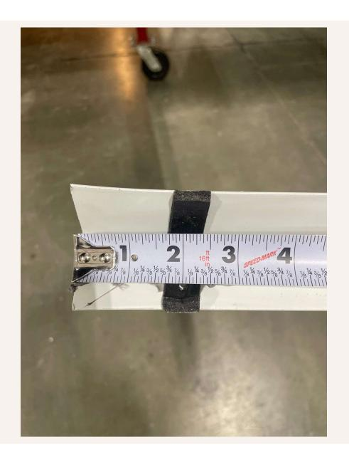
Once you have the rail off add about 3" of 100996 to the end of the rail that will be closest to the inside fascia 1 ¾" from the end. Add butyl tape 101751 to the rail and reinstall it back in place. Insert the screws to secure it you may need to tap the trim with a dead blow to form back to its original shape.
